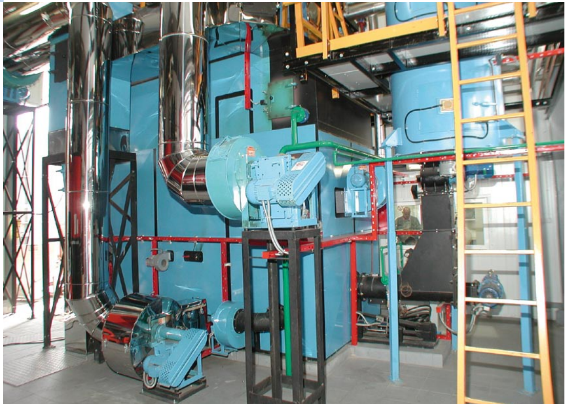
1 MW furnace for incinerating waste timber
