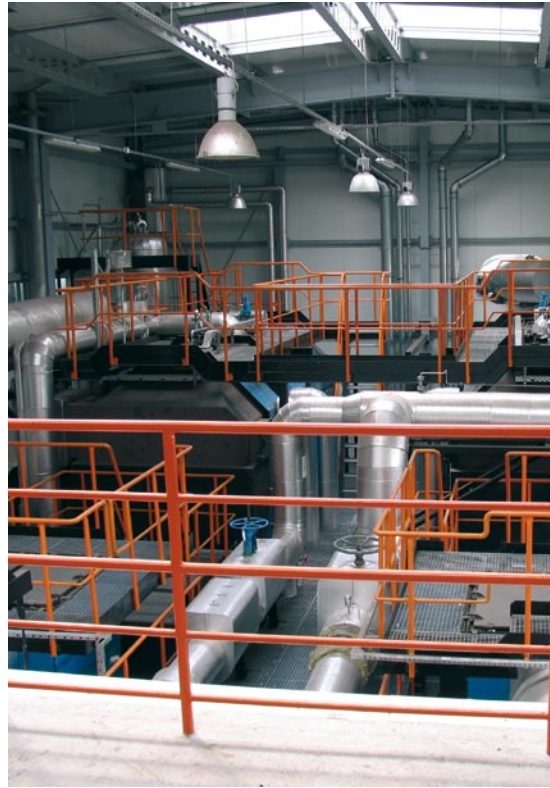
Power plant building (from above)
