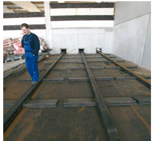
Steel-plated fuel delivery system
