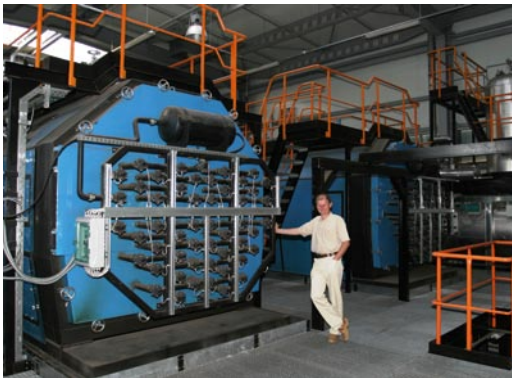
Steam boiler with pneumatic cleaning 32 bar overpressure
