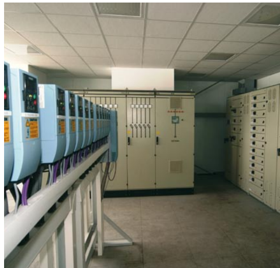
Power plant control system
