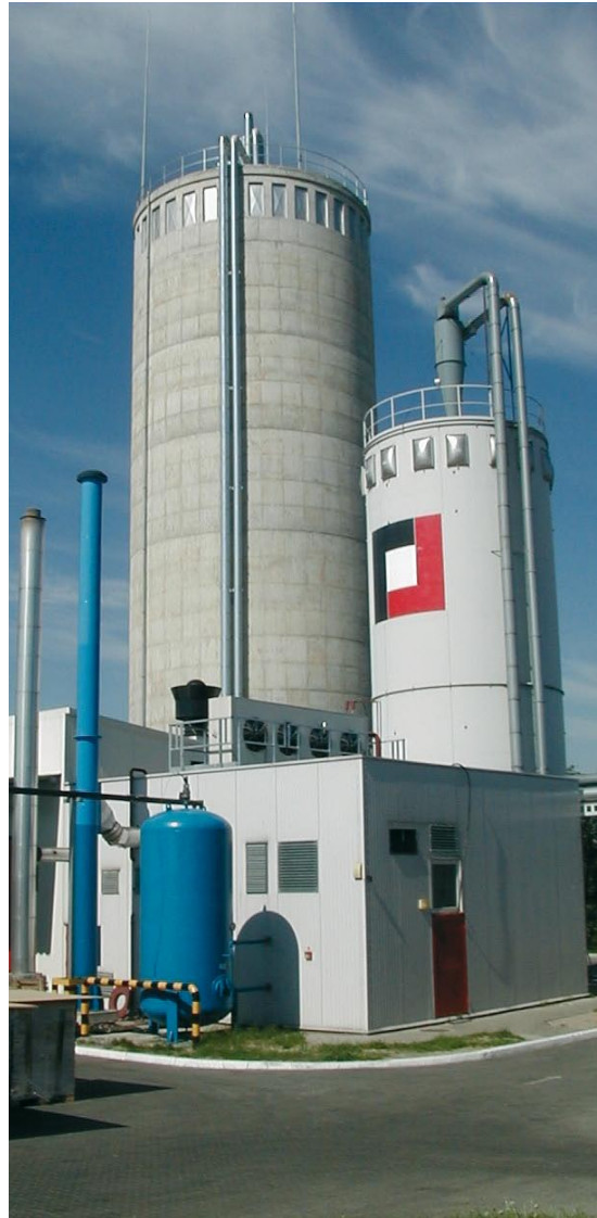
1.0 MW boiler house with silo fuel storage
