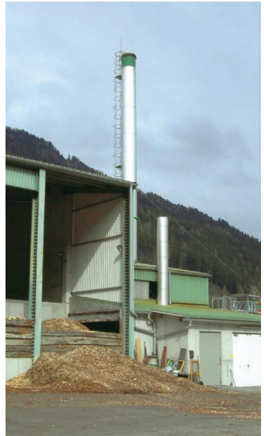
CHP plant in Murau
